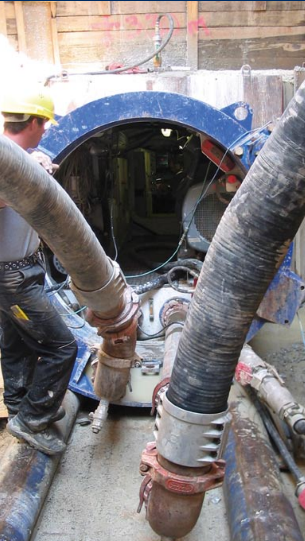
Foto links: Microtunneling
