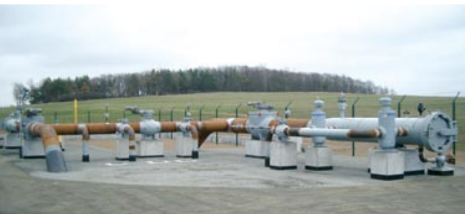
Neue Station Lüptitz
