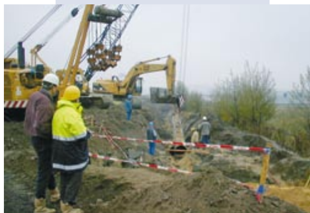
Demontage FGL 216 parallel zur Autobahn
