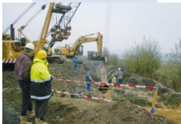
Demontage FGL 216 parallel zur Autobahn
