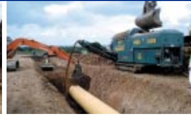
Grading backfill
