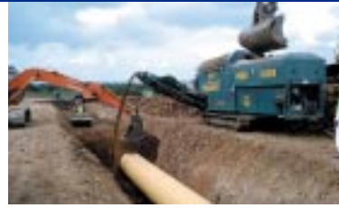
Grading backfill
