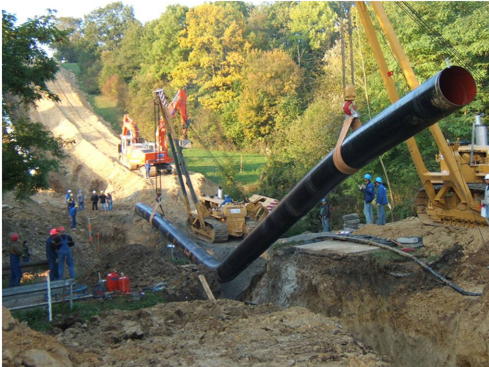
Installation of a pipeline section
